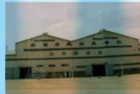
→ Constructed casting plant in Pohang
