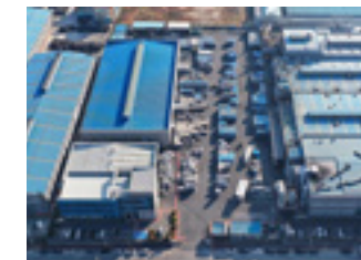
Hyundai Sungwoo Casting (Wheel) Hyundai Sungwoo Casting Co., Ltd. 344 Chungjuhosu-ro(Yongtan-dong), Chungju-si, Chungcheongbuk-do, Korea
