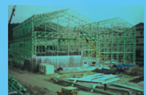
→ Construction site of the 2nd casting plant in Pohang
